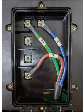
Cable harness diagram FEV-T16/32 (1Ph Connection guide)
