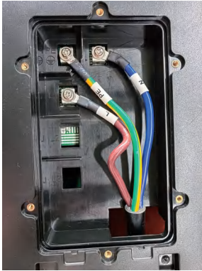
Cable harness diagram FEV-S32(1Ph)
